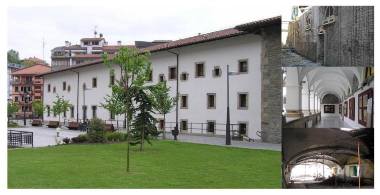
In November 2002, once rehabilitation works were already under way governed by a previous project, the need for substantial changes arose. On one hand, the reason for these changes was based on the structural configuration of the masonry walls and the brick pilasters set on a stone base. On the other hand, the new and considerably higher loads which needed to be transferred to an adequate stratum base given the deficiencies detected in the existing foundation.
